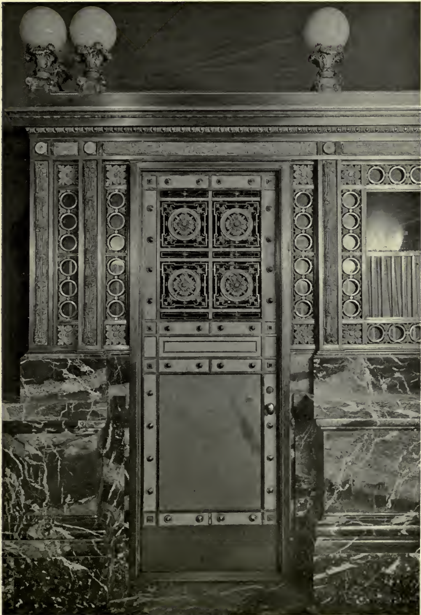
METAL DETAIL IN THE BANKING ROOM.
